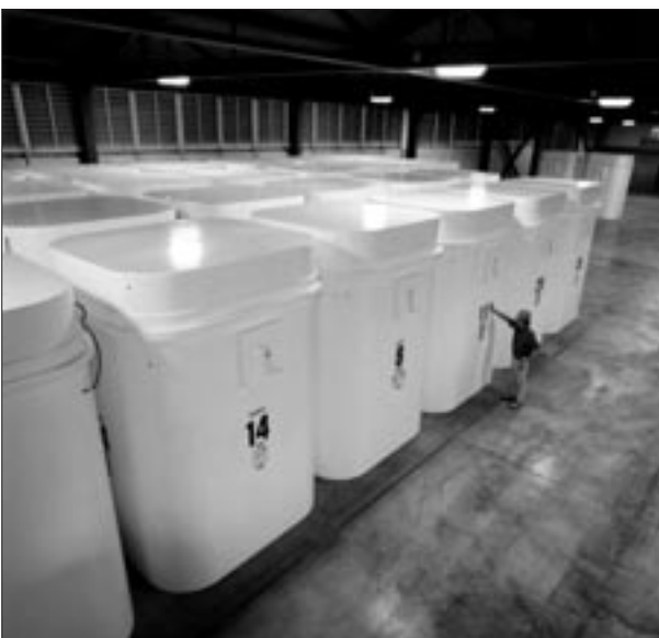
Used fuel dry storage containers stored at Pickering Nuclear, OPG, Canada.
