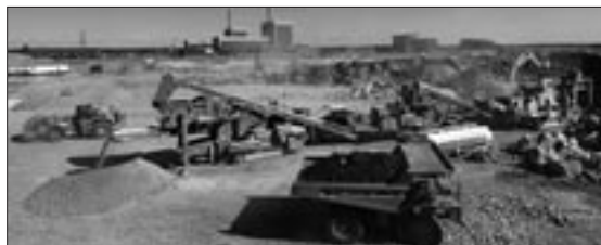
Olkiluoto 3, in April 2004. TVO, Finland.
