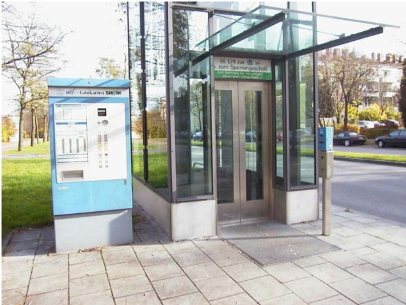
Photo 8. Lift access to U-Bahn, Munich
