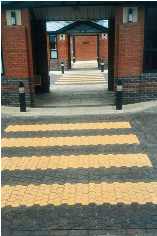
Photo 6. A clearly marked pedestrian way, with dropped kerbs, through a bus station
