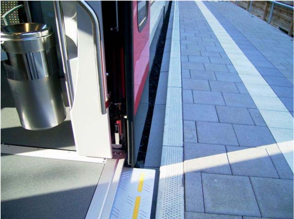
Photo 4. Tactile guidance and platform edge warning surfaces
