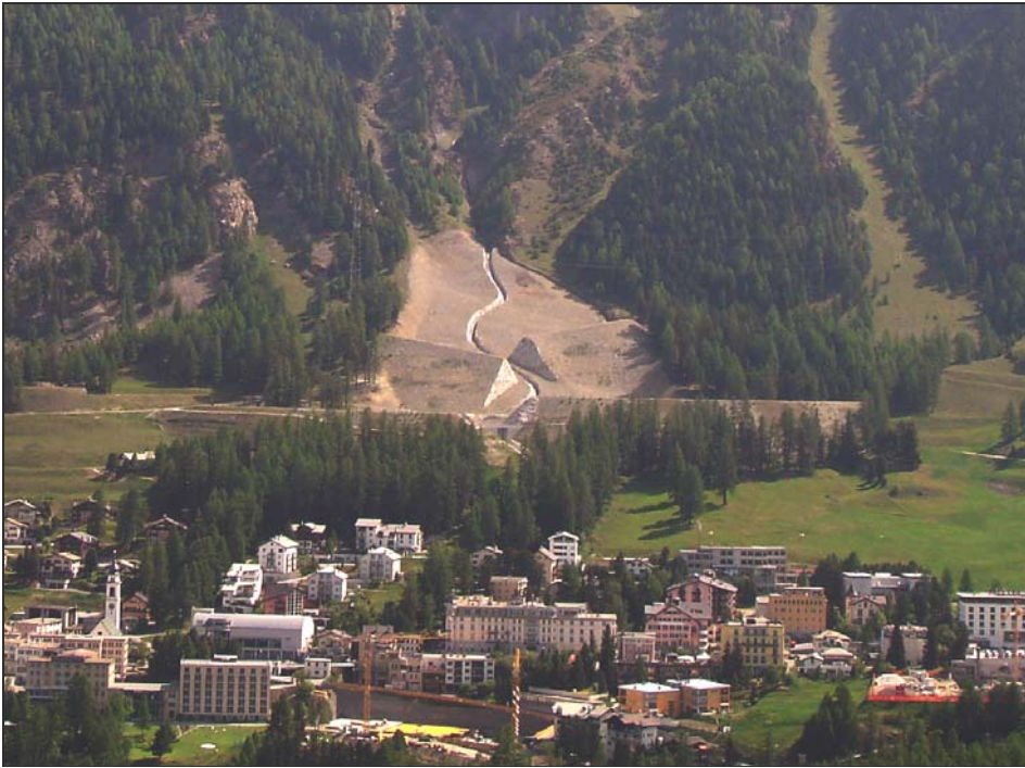
Figure 15. Dams for avalanche and debris flow protection in Pontresina
