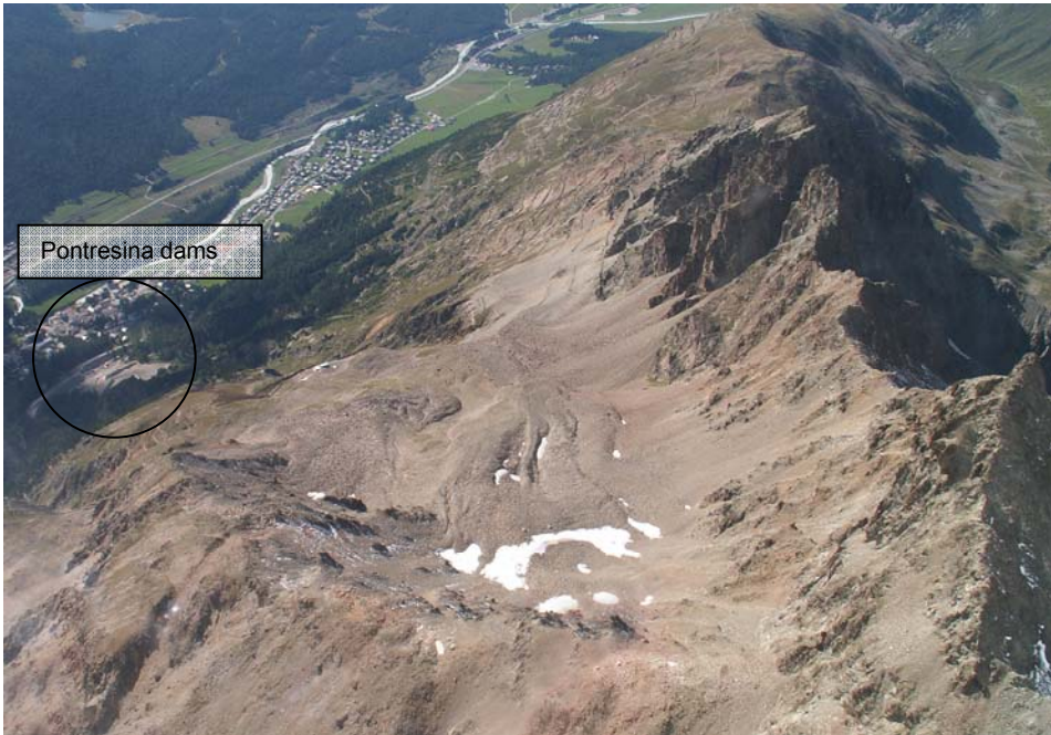
Figure 16. View of the permafrost areas on the Schafberg Mountain above Pontresina
