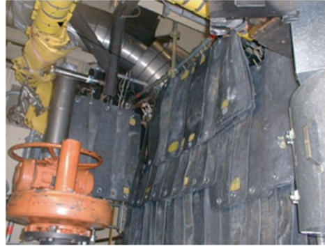
“Bracelet” type protection on a pipe
