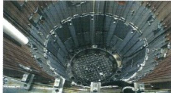
Temporary shielding for replacement for reactor internals (BWR)
