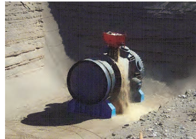
▶ Disposal of the reactor pressure vessel from the Trojan NPP.
