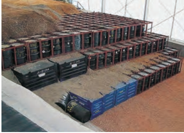
▶ Disposal of very low-level radioactive waste. El Cabril disposal facility, Spain. [Photo: ENRESA]
