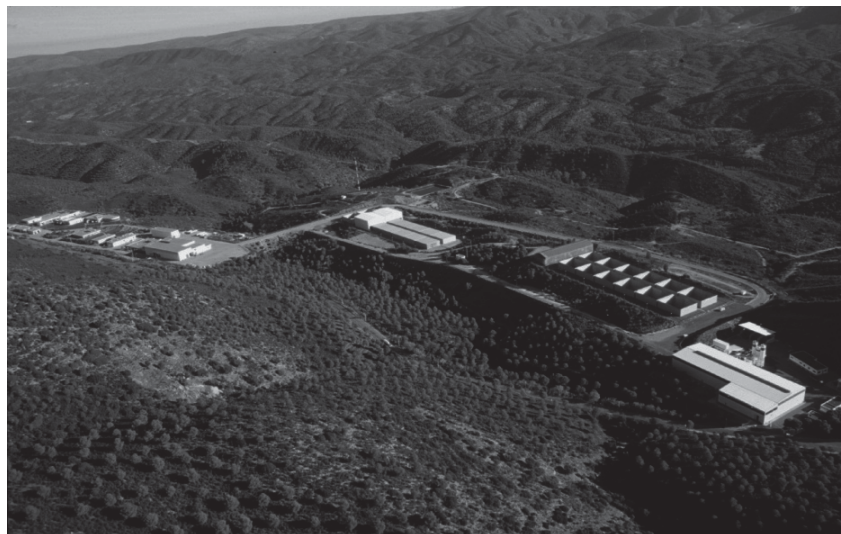
Figure A1.4: Aerial view of El Cabril LILW disposal facility (Spain)
