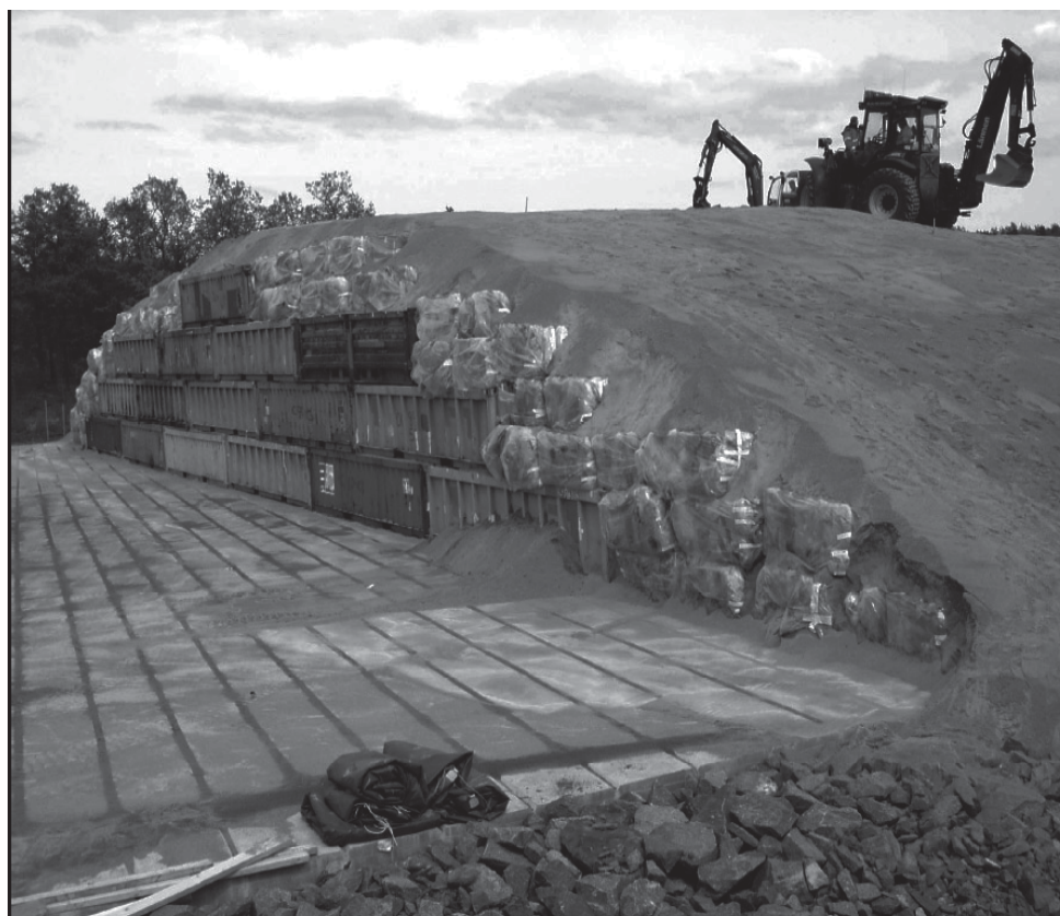
Figure A1.3: Disposal facility for VLLW at the Oskarshamn nuclear power plant (Sweden)
