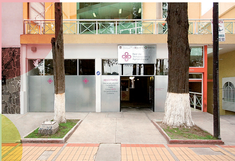
A typical façade: Toluca 2
