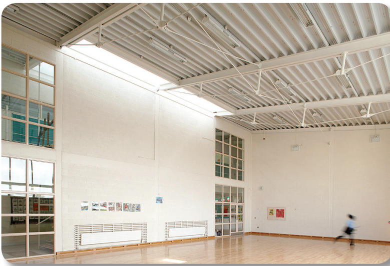
The school hall: balanced glare-free daylight from windows and high-level roof lantern
