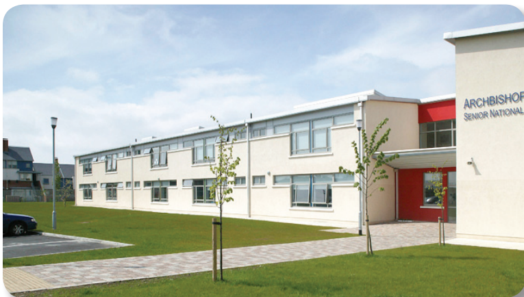
South-facing two-storey classroom block and entrance of first-completed GRD school
