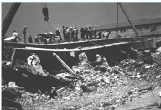
Collapsed General Hospital in Mexico City, 1985
