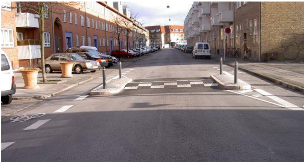
Figure 5.21 Road hump with kerbed islands and bollards
