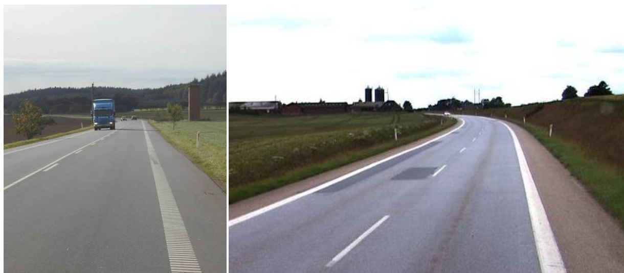
Figure 5.20 Paved shoulders on rural roads (Denmark)
