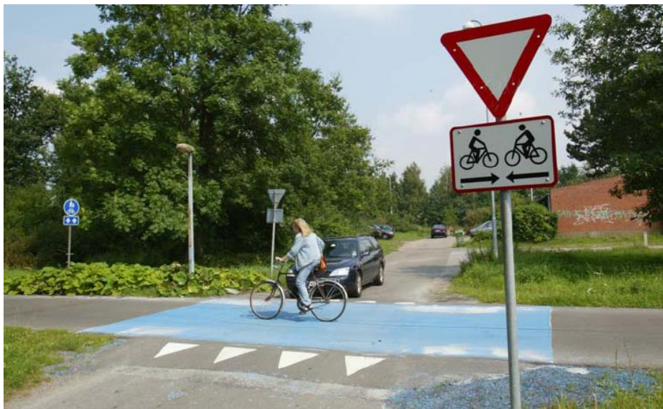
Figure 5.25 Bicycle crossing on raised plateau and with right of way for bicyclist (Denmark)
