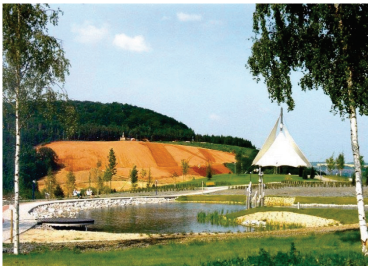
Figure 3.2. The spa park at the Schlema site (Aue), with reshaped, covered and re-cultivated waste rock piles in the background
