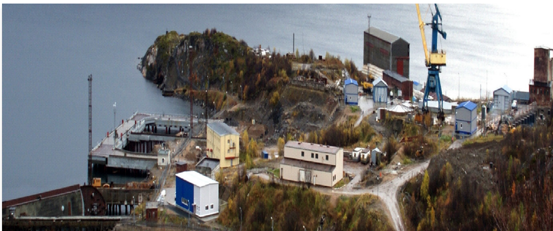
Figure A2.8. General view of the technical territory of the Andreeva Bay site
