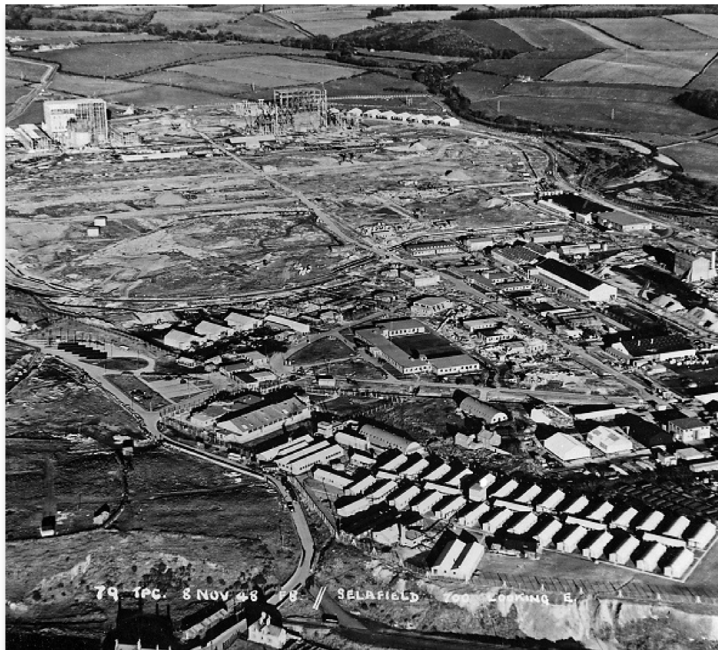
Figure A2.2. The site with facilities under construction in 1948
