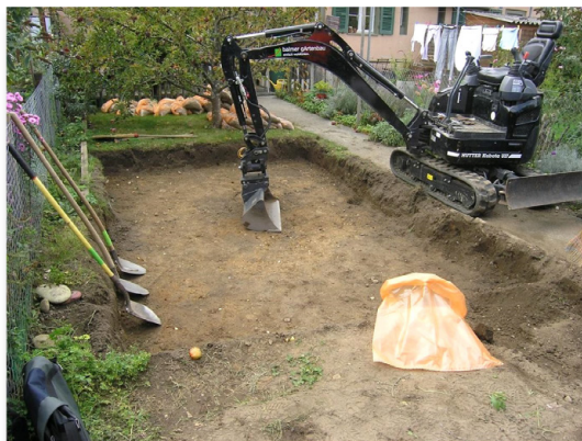
Figure A3.18. Excavation of radium-contaminated part of a garden
