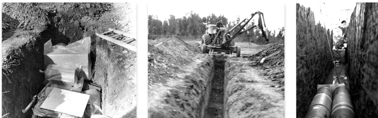
Figure A3.3. Excavation and filling of trenches at LFLS
