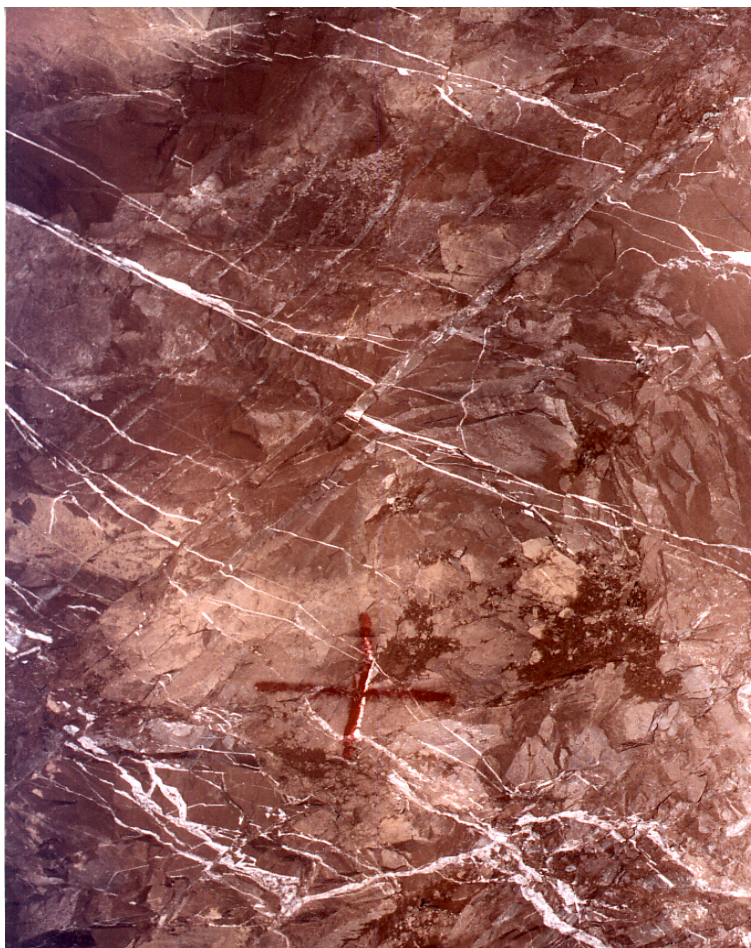
Figure A3-37: Tectonic joints on the wall of the URL exploration tunnel filled with calcite veins
