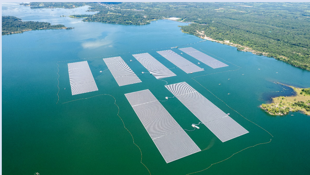
Figure 11 Floating solar projects at Sirindhorn Dam, Thailand
