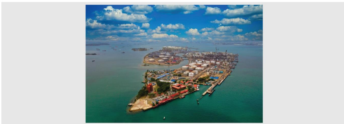
Figure 4.5. Shell is building a chemical recycling plant in Singapore
