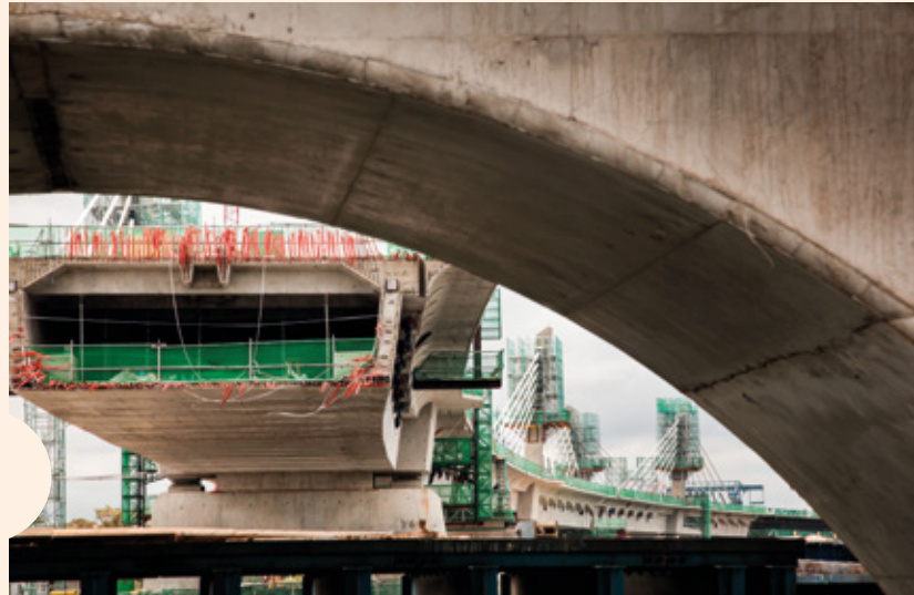
Construction of the Kazungula Bridge, linking Botswana and Zambia.
